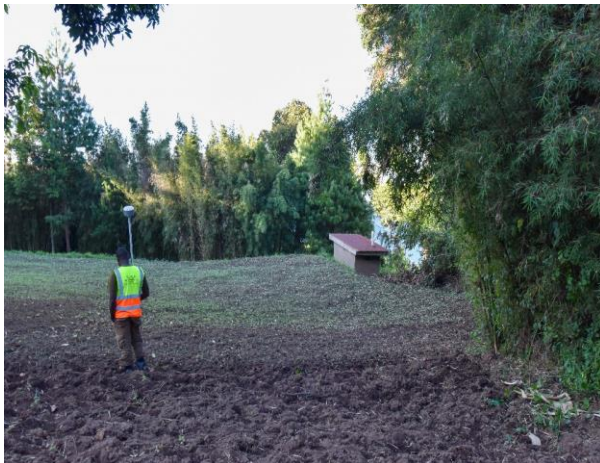
Land surveyor carrying out survey at site
