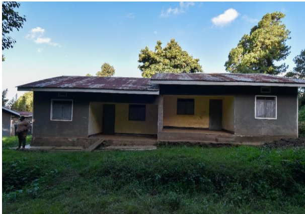
Staff and Patrol house to be renovated at Echuya site
